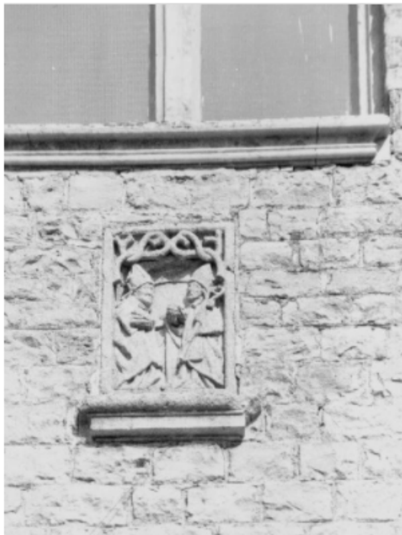
[© KIK-IRPA, Brussels (Belgium), cliché M250680]
